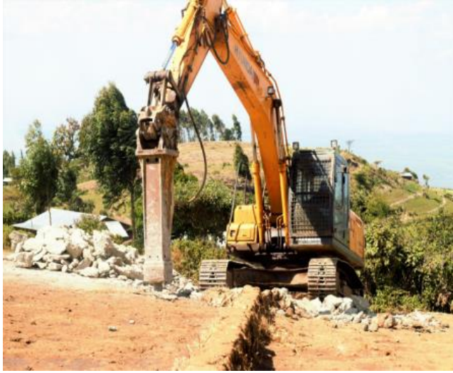
Figure 9.a Breaking Rock on Cheminy-Atar Road in Kween District, where Major Rocky Sections
