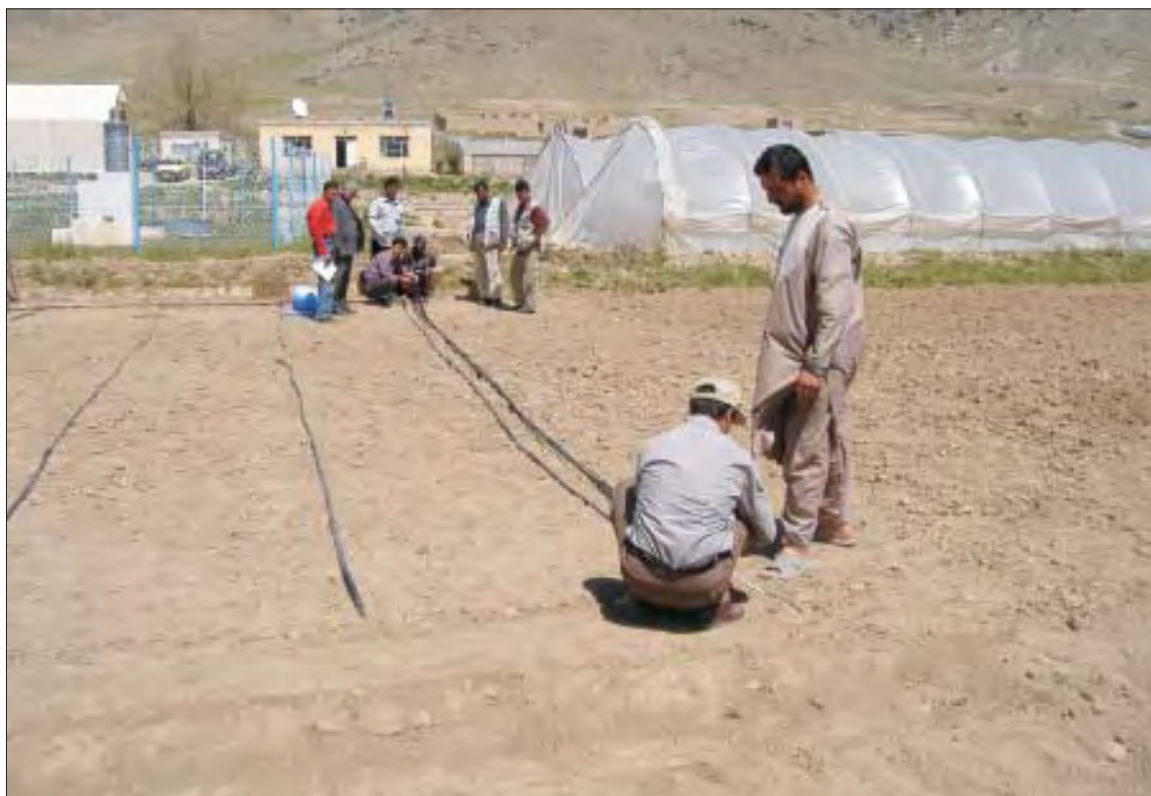
IFDC and MAIL staff placing drip tubing for the bucket drip system at the Quargha Research Station, Kabul, Afghanistan.
